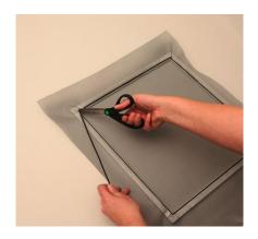
• When your reach the end of the 4<sup>th</sup> side cut the spline with a pair of scissors and push the end down into the corner.
